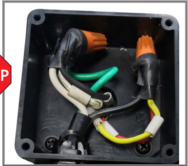
Figure 129. Motor wiring at 120V.
