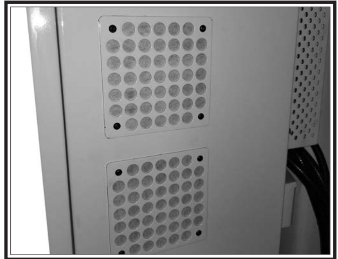
Figure 41. Air filter external covers.
