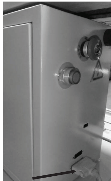
Controller cable fitted to cabinet socket
