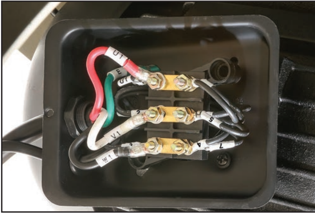
Figure 167. Motor wiring (220V).
