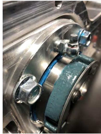
Grease Coming Out The Front Seal
